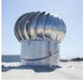
Rooftop Turbine Vents
