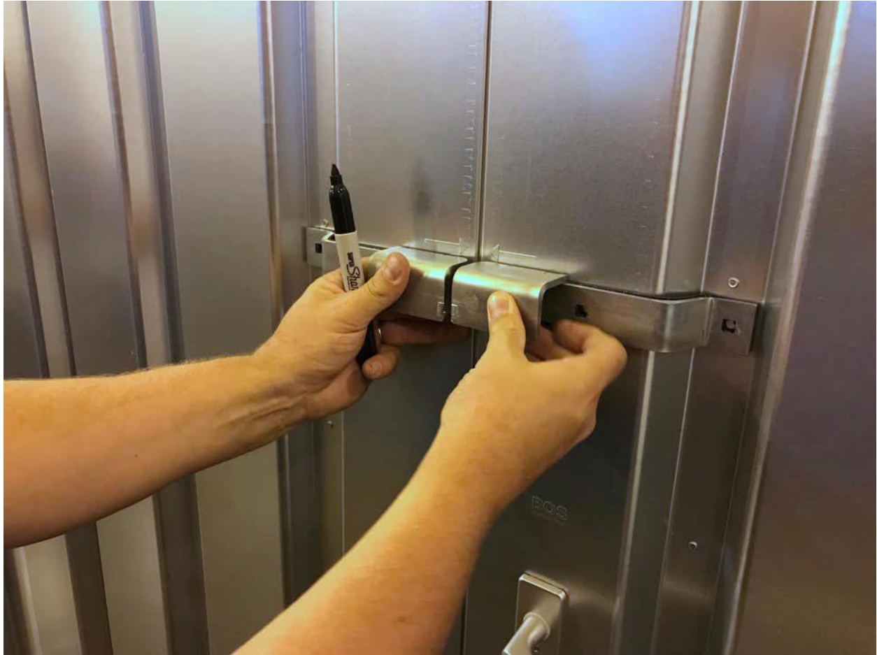
Finishing the marking of the holes.
