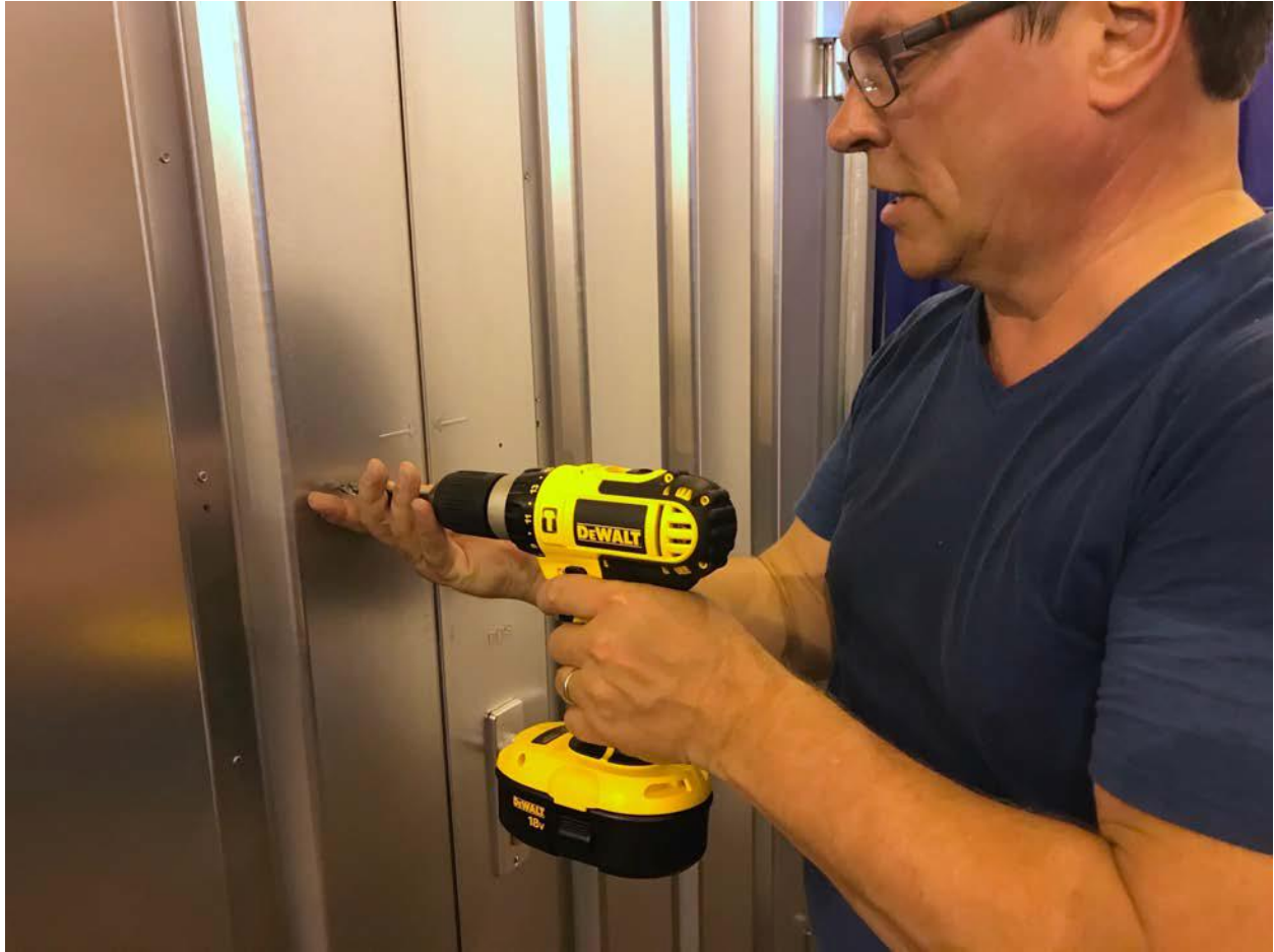
Drilling the holes
