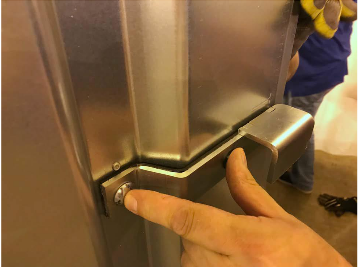
Installing the hardware.
