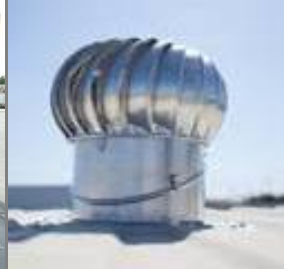
Rooftop Turbine Vents
